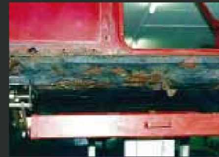
Not only were the inner and out sills shot, but check out the effect of the wood on the bodywork.
